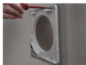
Fixing of the internal grid's support
