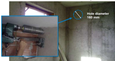
Placing of the duct
