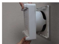
Placing of the fan unit on the support
